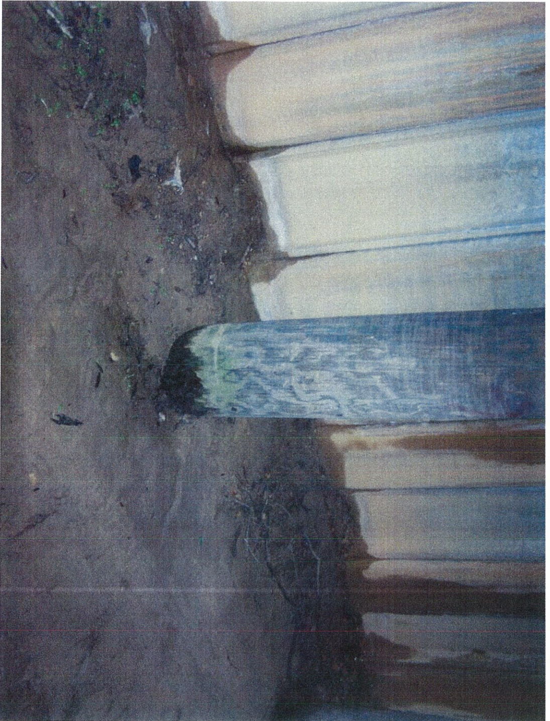
Timber pile typical
